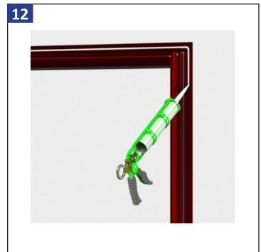
Apply a 3/8" diameter bead of sealant along the interior side of the flashing flange.
