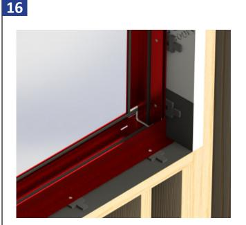
Square, plumb, and level the flange fin system into the opening shimming as needed at each fastener location.
